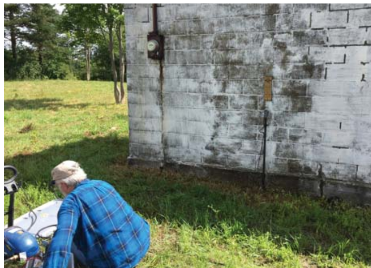
Tom Joneson getting ready to power wash the building.
